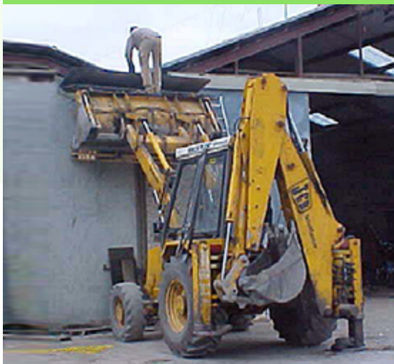
► Figure 34. Unsafe practice when working at height as there is no fall protection in place.
