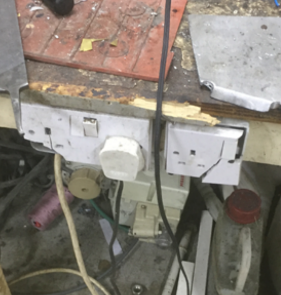
► Figure 49. Damaged electrical sockets.
